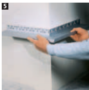
Corner of building Use Sto Universal Starter Track Corner Profiles at external corners of buildings. These profiles adapt to the angle of the corner. The Sto Universal Starter Track Round is used for curved elements on buildings.
